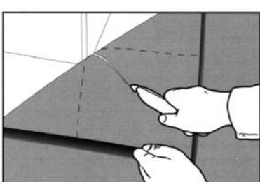
When fitting an out-corner, the sheet is folded against the corner and cut about 5 mm ( 1/4 in.) from the floor. The guidelines in the picture show the corner on the sheet and the position of the cut at about a 45- degree angle. Then a diagonal cut is made as shown.
