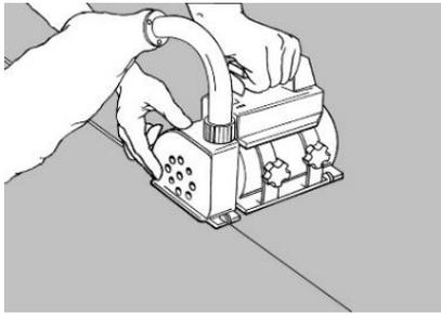
The sheets are heat welded. Do not weld until the adhesive has bonded completely. The joints are chamfered or grooved to about  $\frac{3}{4}$  of the thickness using a hand grooving tool or machine prior to welding.
