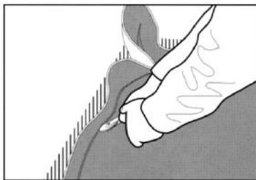
Use a Hockey Stick or Corner Roller to press the material firmly into the juncture between the floor and wall. In areas where one sheet is sufficient to cover the subfloor, the adhesive can be applied over the entire surface area before installing the sheet.
