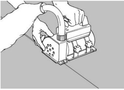
The sheets are heat welded. Do not weld until the adhesive has bonded completely. The joints are chamfered or grooved to about  $\frac{3}{4}$  of the thickness using a hand grooving tool or machine prior to welding.
